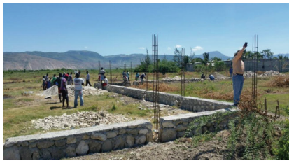
Orphanage Perimeter Wall Build Began - August 2016
